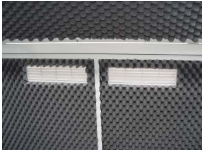
Sound proofing inside walls
